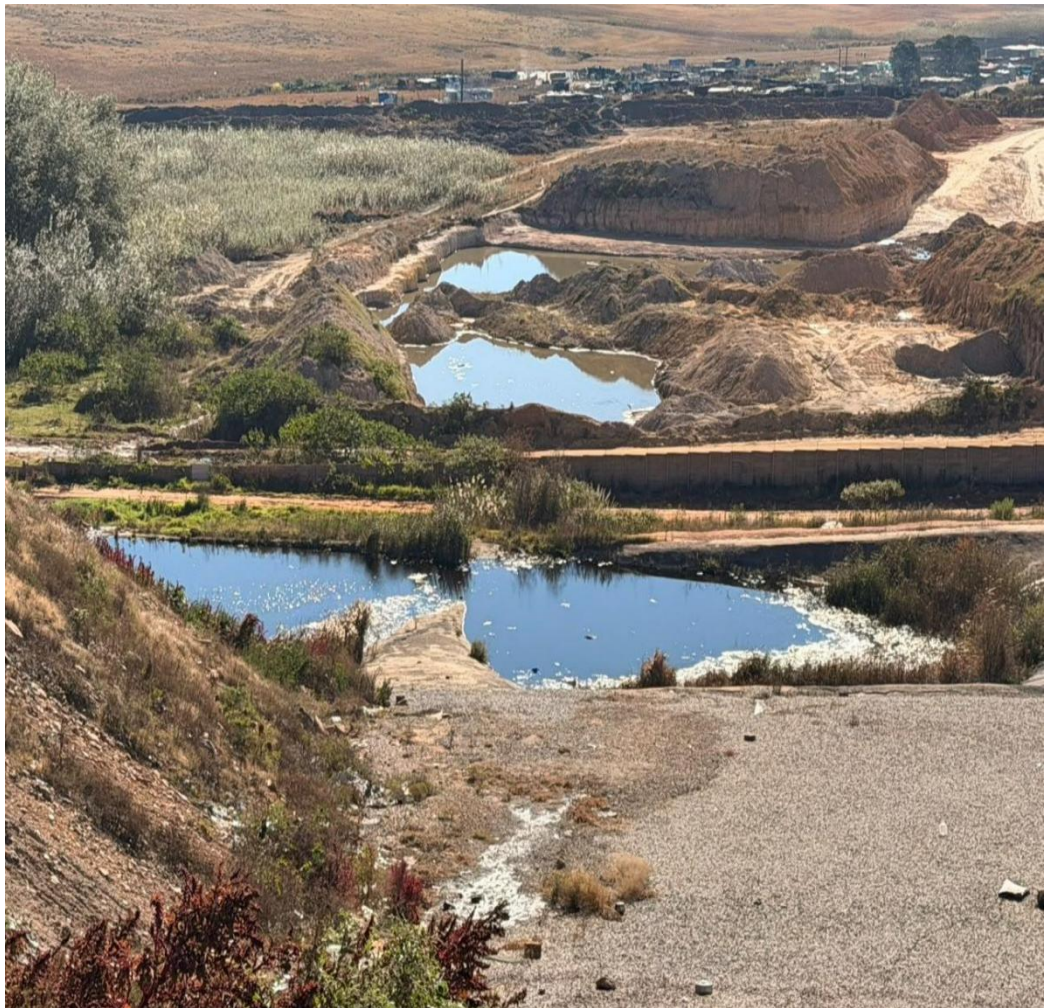
Figure 10; Leachate pond and leachate leaking to the nearest gathered water
