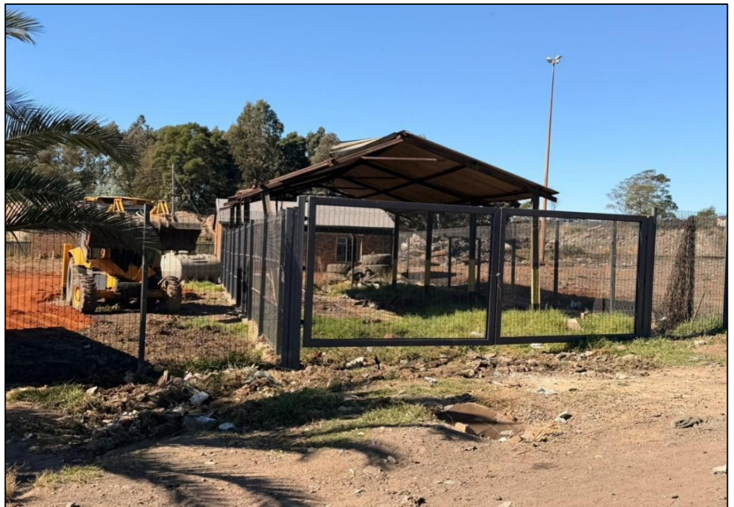
FIGURE 4: Fuelling and workshop area
