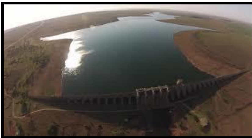
Figure 7: Photo of Middelburg Dam
