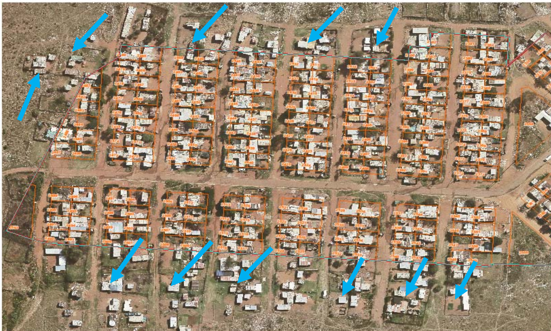
Source: STLM Geographic Information System – GIS, Part of Newtown to indicate extra shacks outside legal boundaries of stands: The image for only use to indicate the surrounding situation in Newtown.
